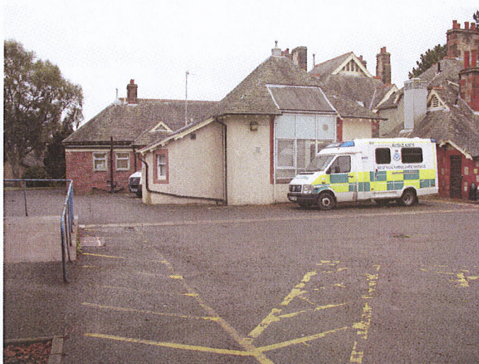
Figure 6.1: Extensions to the rear of the listed Victoria Infirmary building
