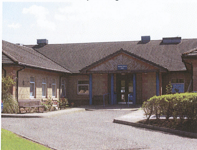
Figure 6.3: Front entrance of the Jeanie Deans Unit building to the south east of the Victoria Infirmary building
